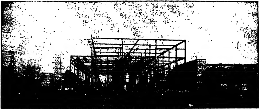
The 60,000 Volt (outdoor) and 12,000 Volt (indoor) Switching Stations at Echota, Niagara Falls Power Co.
